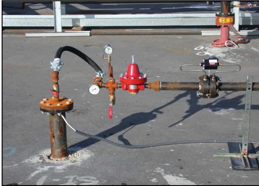
Figure 4.3 Steam Injection Well Equipped with Pressure Regulator and Metering
