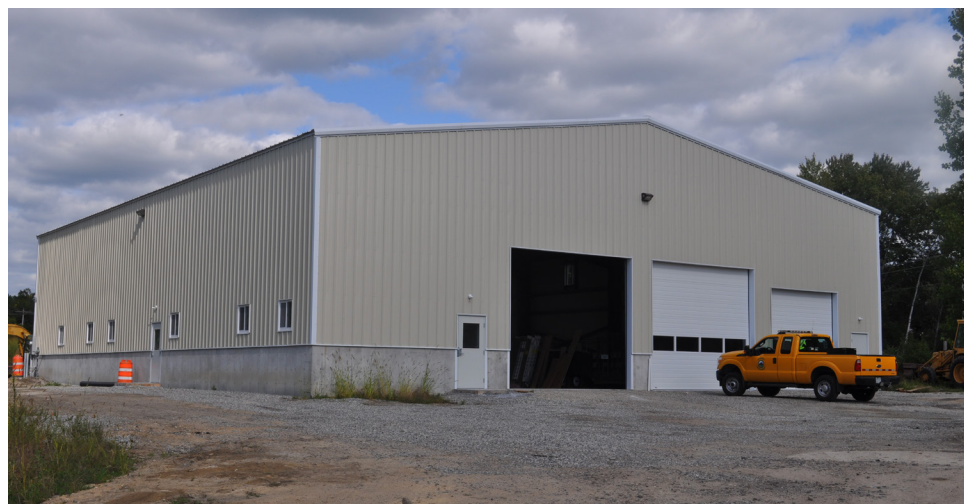
Above: The new public works building
