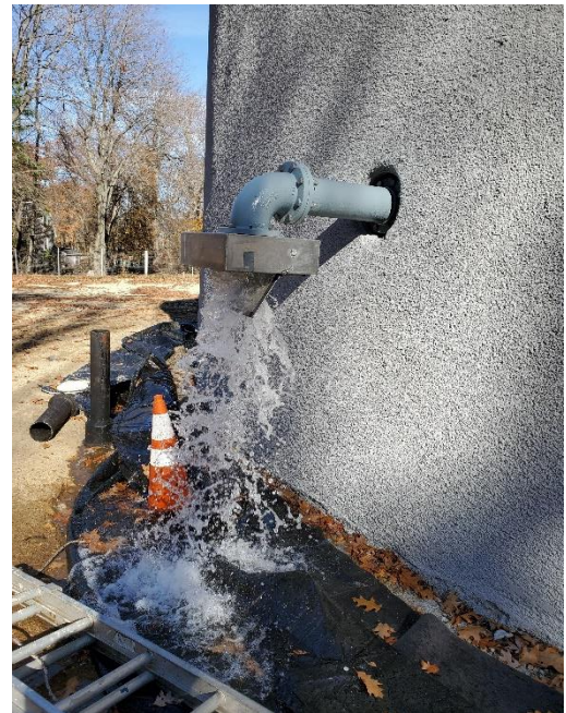
Figure 4: The tank overflow during filling.
