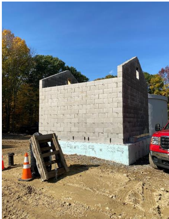
Figure 3: Valve Building Unit Masonry
