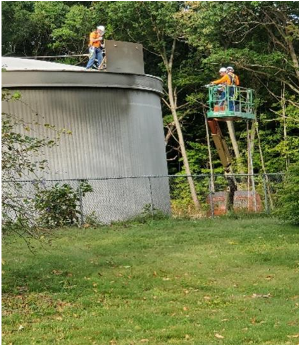
Figure 5: Contractors spraying shotcrete on the tank.
