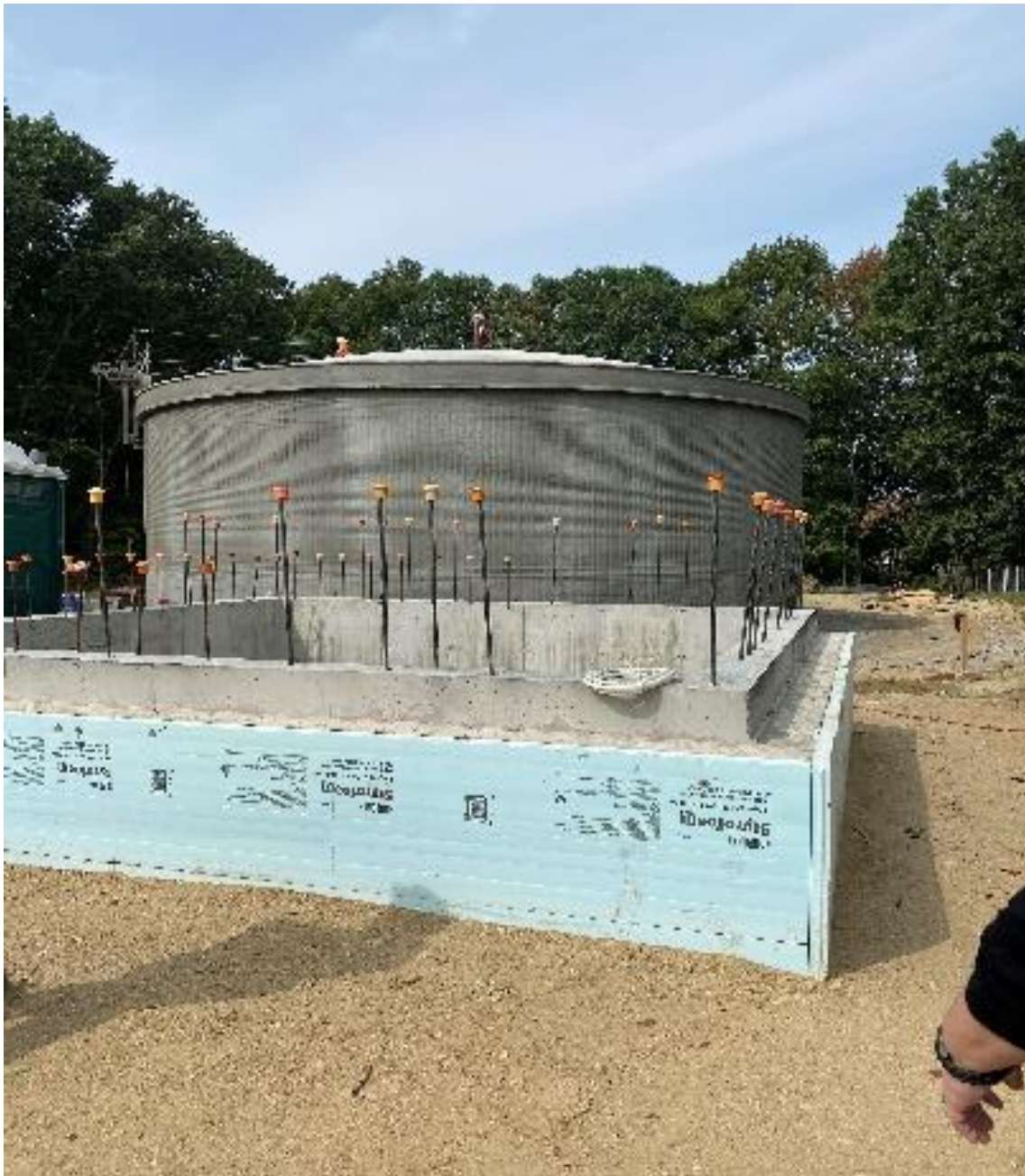
Figure 4: The water storage tank and valve building foundation.
