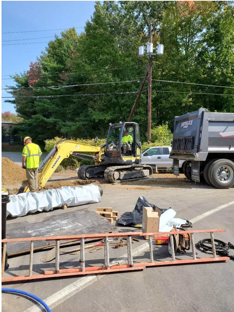
Figure 2: The contractor is beginning to install watermain on Hale Spring Road.
