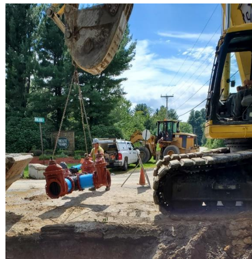
Figure 2: Installing PVC watermain.
