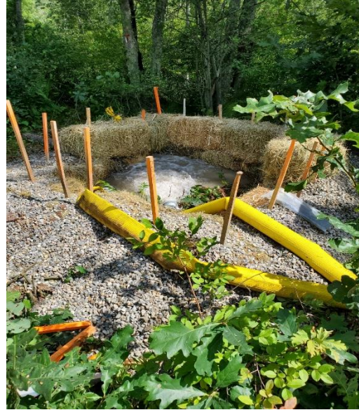
Figure 4: Dewatering at the pump station.
