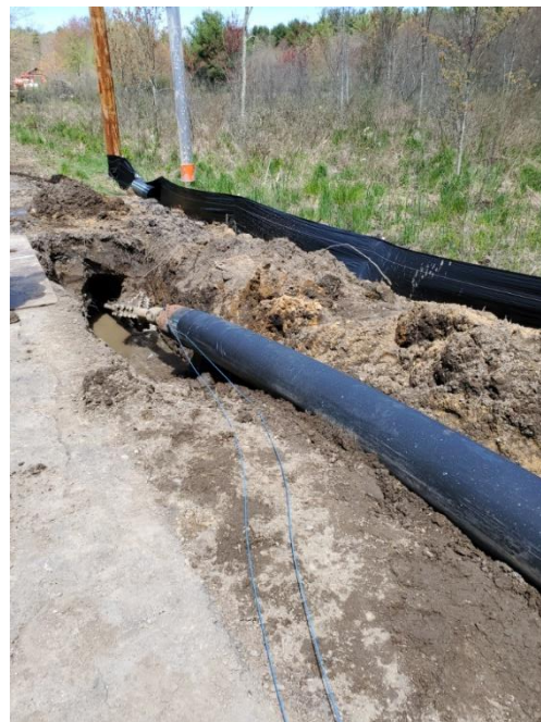
Figure 2: Directional Drill under Bryant Brook
