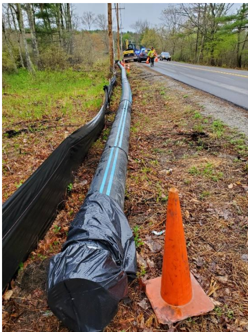
Figure 1: Pipe Prepared for Directional Drill
